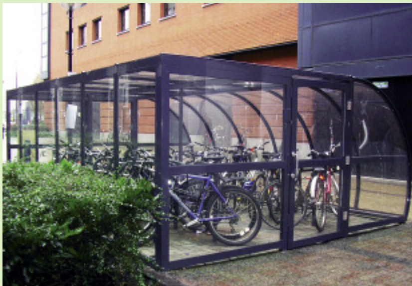
The new shelter outside the Geoffrey Manton Building has space for 20 cycles.
